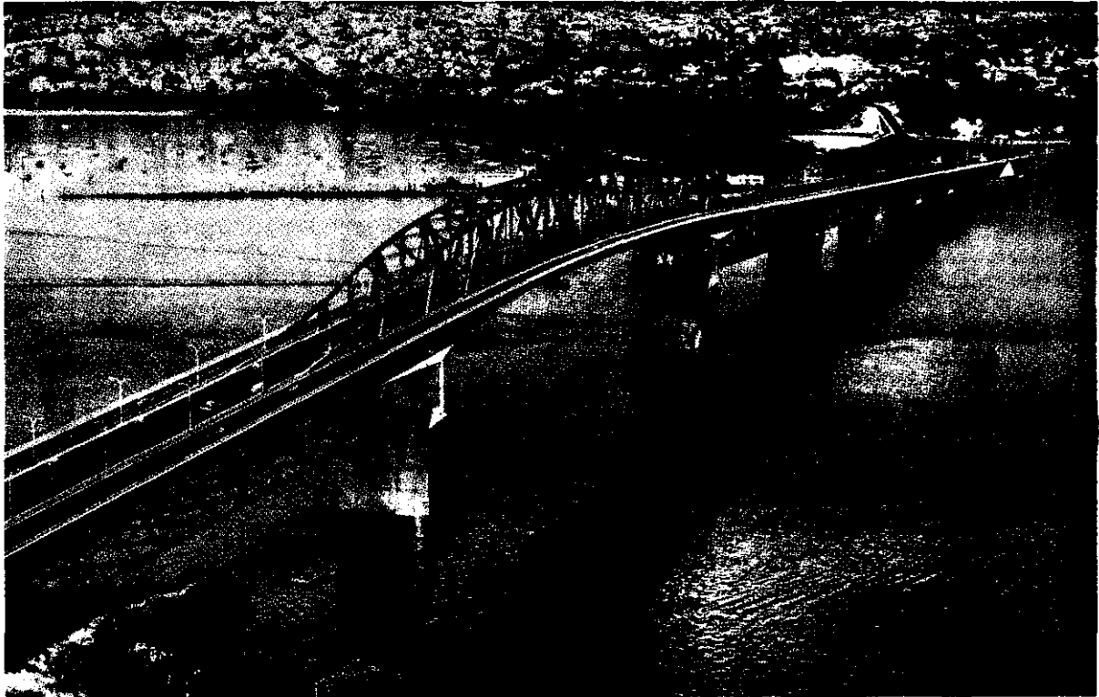
Fig. 1. The existing Auckland Harbour Bridge, with an artist's impression of the new structure superimposed.
